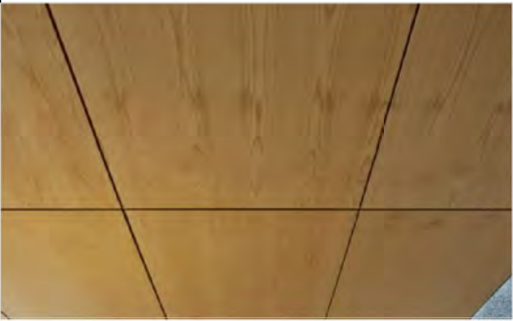
SPLAYED ROOF FEATURE - 'SGI ARCHITECTURAL - PRODEMA' COMPOSITE WOOD PANEL (TP)
